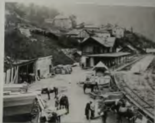
Construction site of the railway line.
