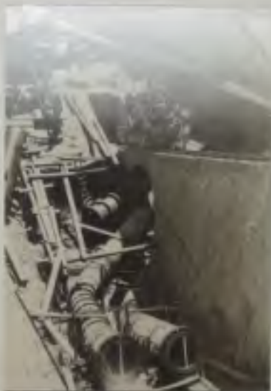
Large pipe or tunnel boring machine at the construction site of the railway line.
